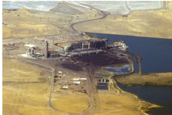
Figure 5-29 Four-Corners Power Plant, New Mexico, U.S showing 3 main clusters of stacks. From left to right, starting with the tall stack (cluster #1): Clusters #1 - #2 separation ~ 400 m; Clusters #2 - #3 separation ~ 150-200 m.
